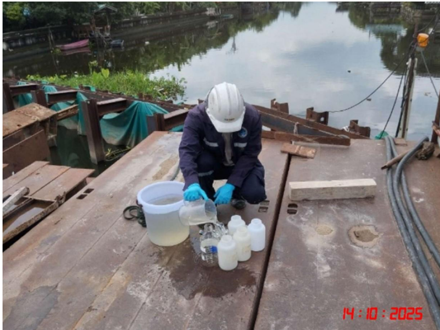
Water Quality Monitoring by Mine Engineering Consultant Co., Ltd. Mahasawat Canal Water Transmission Tunnel Construction Project
